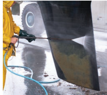
A slime layer is easily removed with a water blast.
