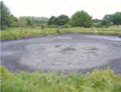
Farm anaerobic pond: The bubbles indicate good biogas activity which can be captured and used to reduce greenhouse gas emissions.
