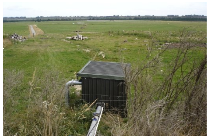
Figure 2: Existing irrigation pump house
