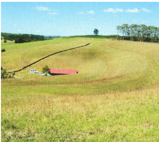
Figure 3: Manuwai Dam (downstream side)
