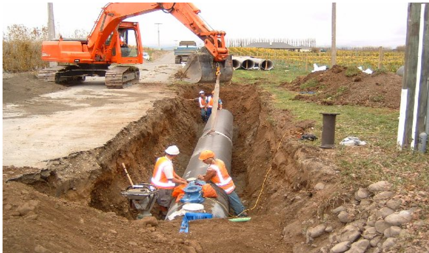
Figure 4-3: Laying Pipes for Southern Valleys Irrigation Scheme
