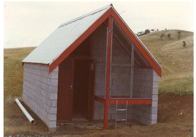
Figure 2: Wainuioru RWS staging site pumpstation
