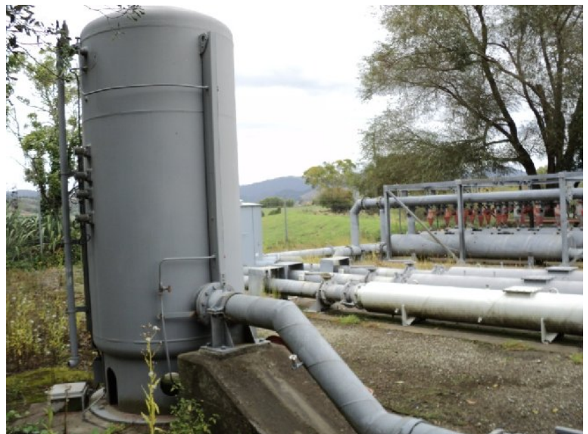
Figure 3: Headworks (sediment removal, pumps, break pressure tanks)
