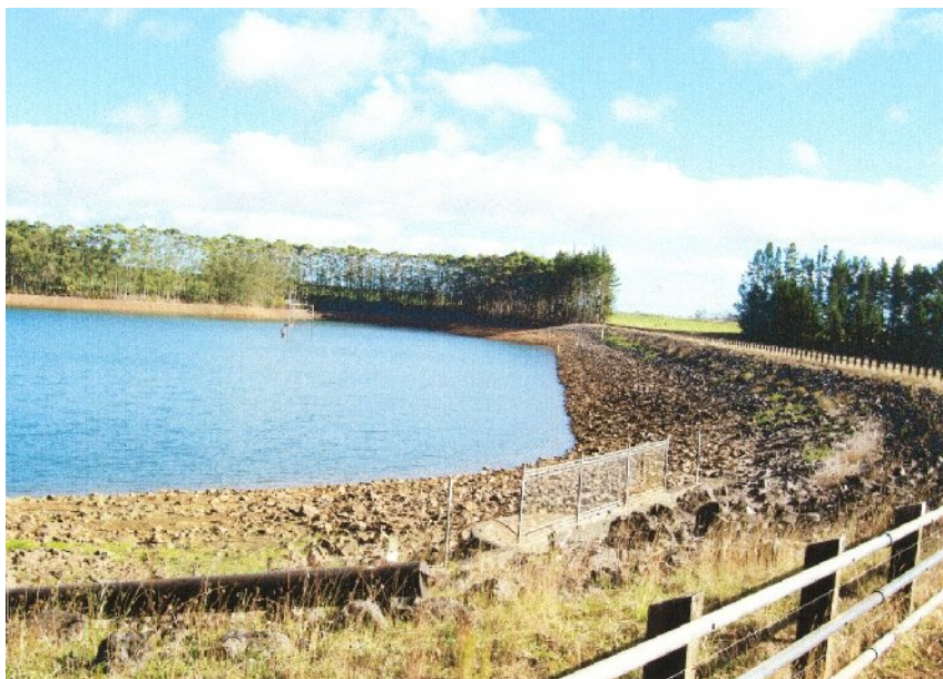
Figure 6-2: Waingaro Dam at Kerikeri Irrigation Scheme
