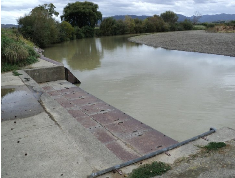
Figure 4-2: Otara River and Intake Structure for Tablelands Irrigation Scheme
