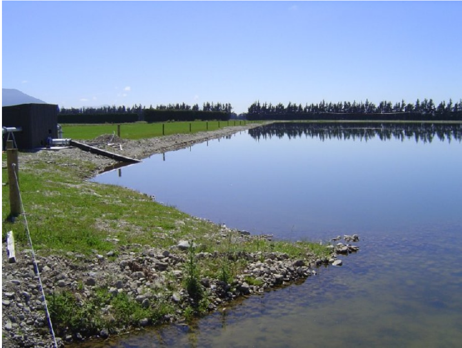
Figure 4-5: Storage Pond at Waimakariri Irrigation Scheme
