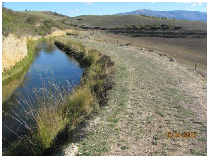
Figure 4-1: Main Race at Manuherikia Irrigation Scheme
