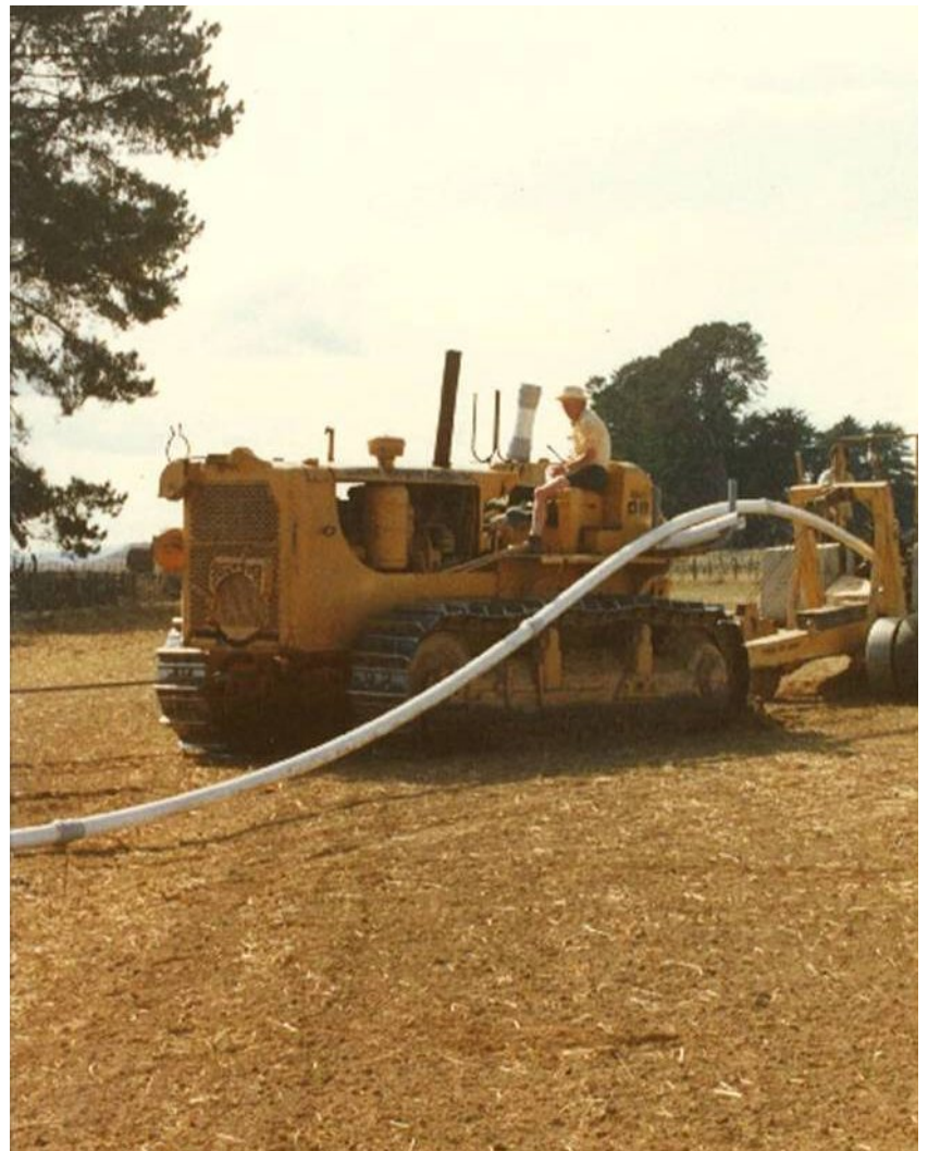
Figure 4: Hunterville RWS pipeline installation
