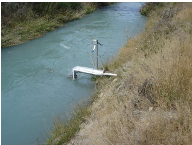
Figure 4: Existing irrigation pump offtake
