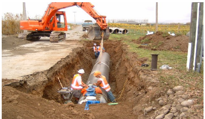
Figure 3: Laying pipes for the irrigation scheme
